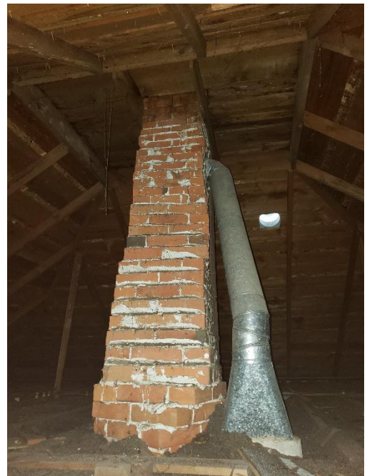
Hipped roof framing with a central brick chimney.
