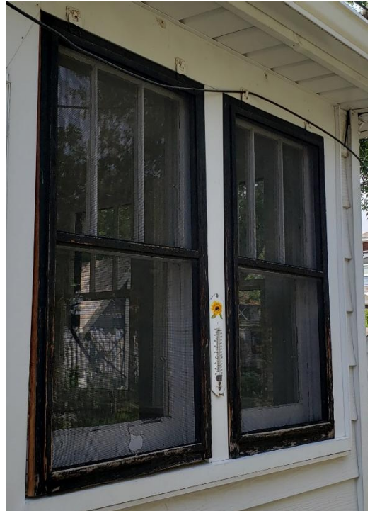
Wood framed screens on mudroom windows.
