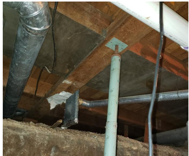
Steel column supporting a flat wood beam.
