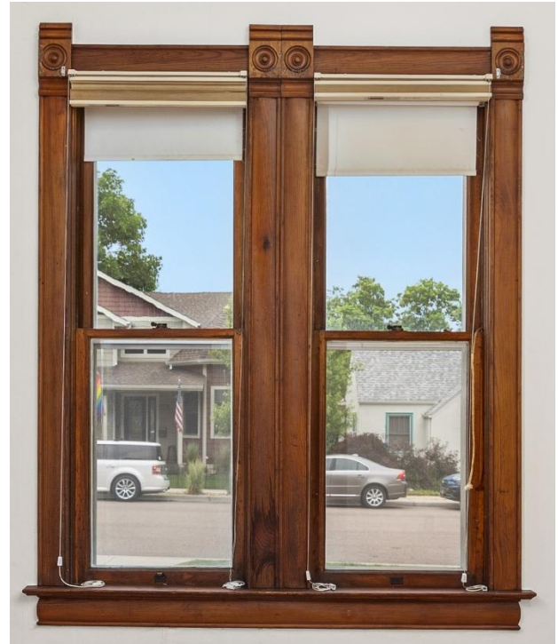
Original wood windows with counterweights.
