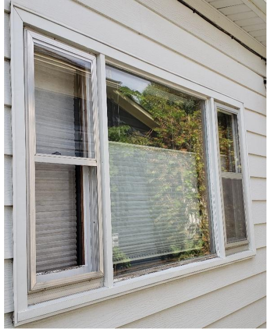
Replacement windows and aluminum storm windows.
