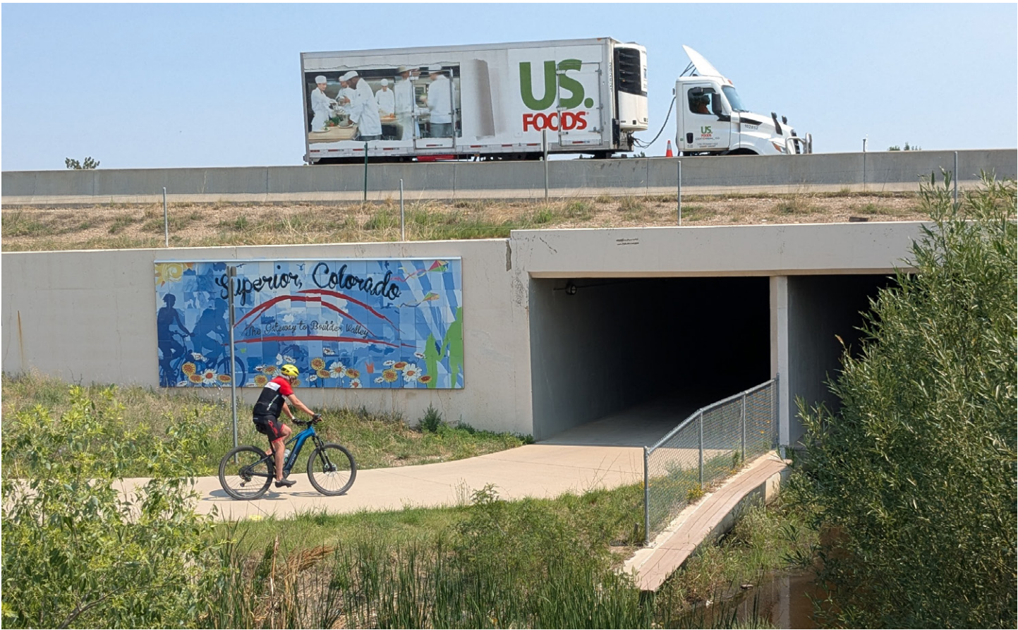
Trail through Underpass (Credit: PROS Staff)
