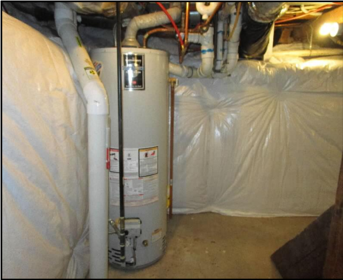
1016 Main St. CRAWL SPACE/MECH
