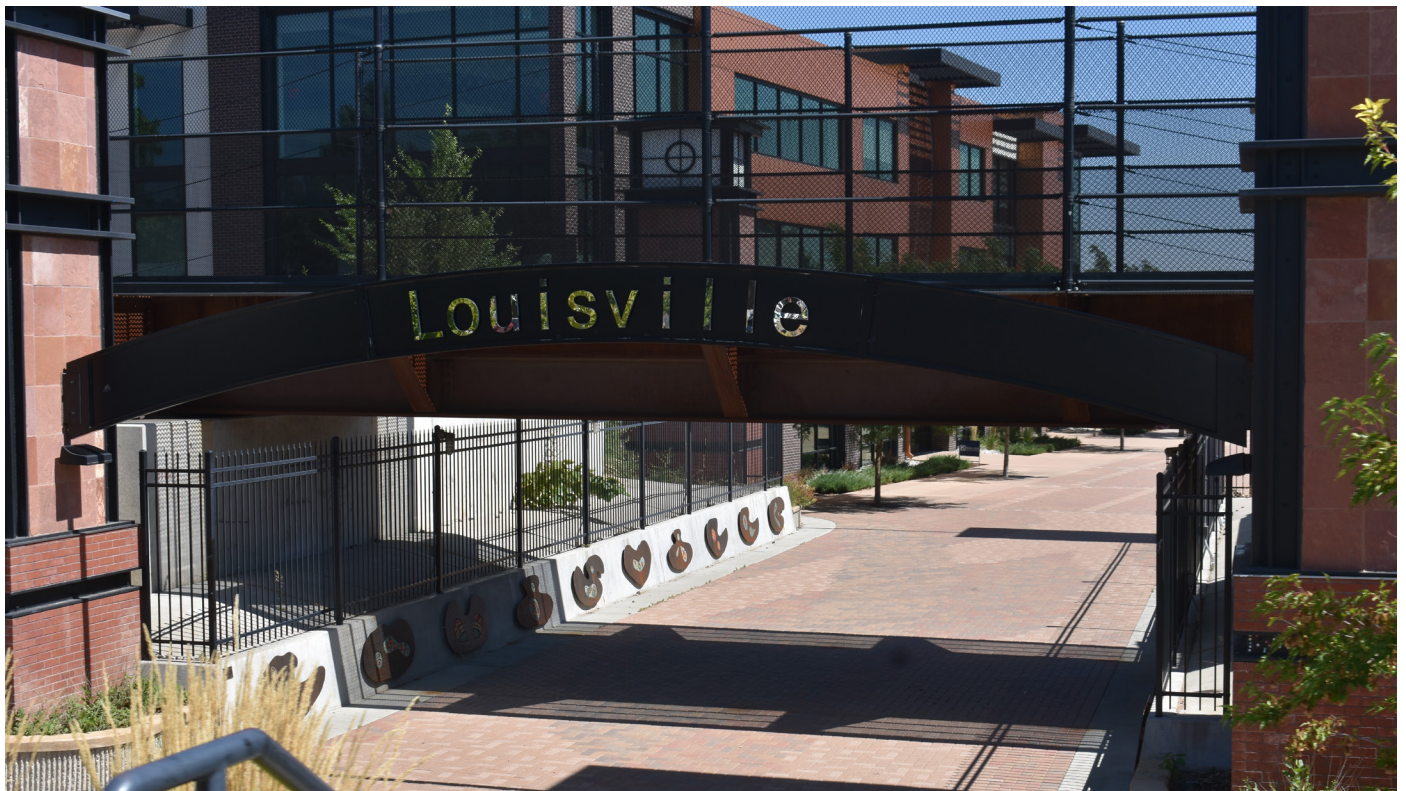
Louisville Bridge Source: DesignWorkshop
