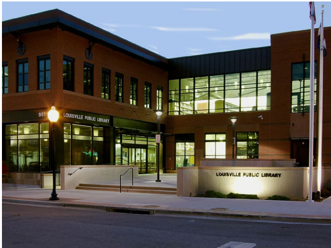
1 Louisville Public Library (Source: Louisville Public Library)
