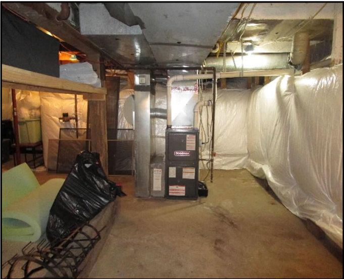
1016 Main St. CRAWL SPACE/MECH
