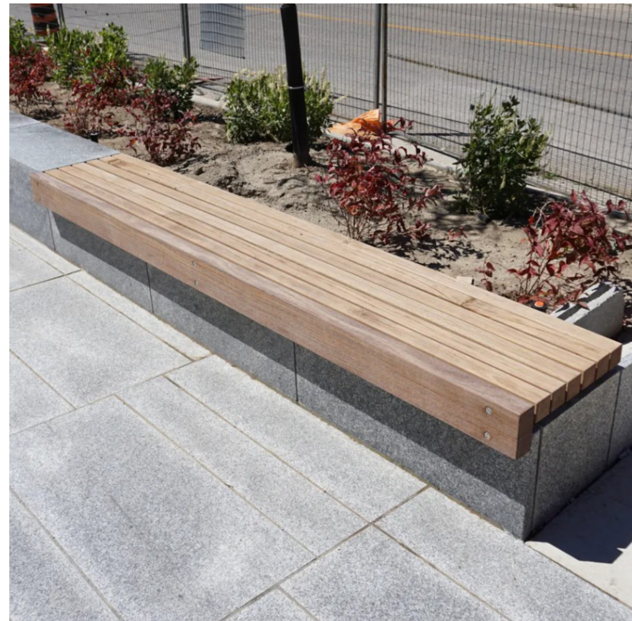
CONCRETE SEATWALL W/ WOOD BENCH
