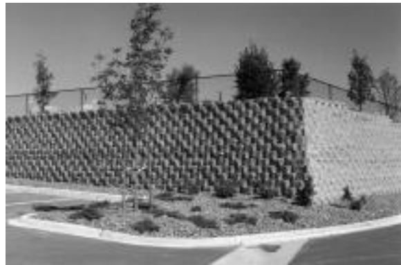
6.1.A - AVOID RETAINING WALLS IN EXCESS OF 30"
