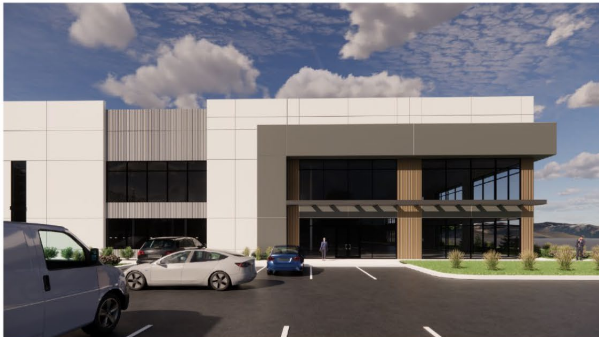
Long side of building facing a street, corner entry feature
