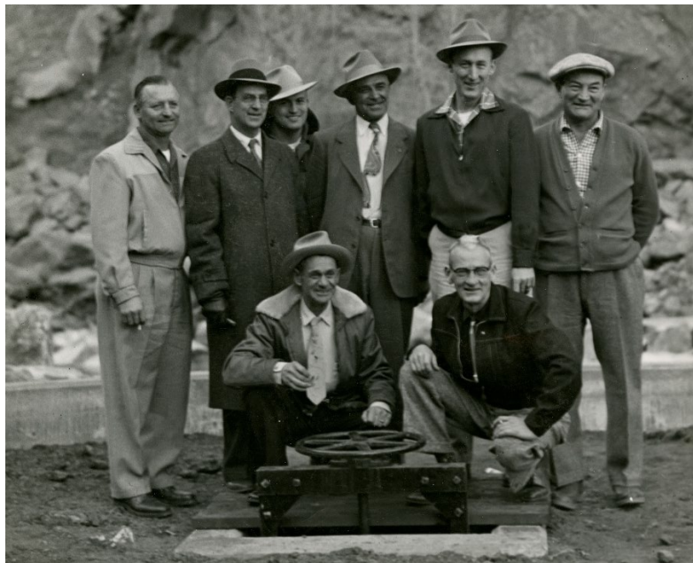
Ring Dionigi (front left) during the dedication of the pipeline in Eldorado Canyon to improve Louisville's water supply in 1956.
