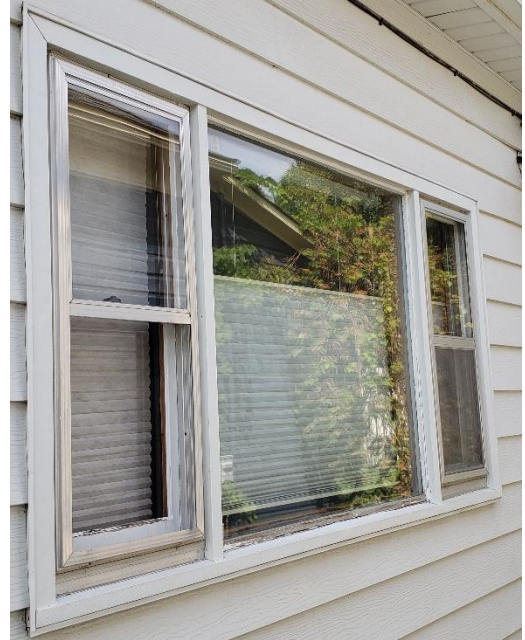
Replacement windows and aluminum storm windows.
