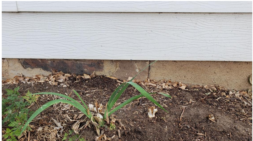
Exterior view of transition from stone foundation (left) to concrete foundation (right).
