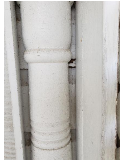
Original wood shiplap siding behind metal siding and an attached column.
