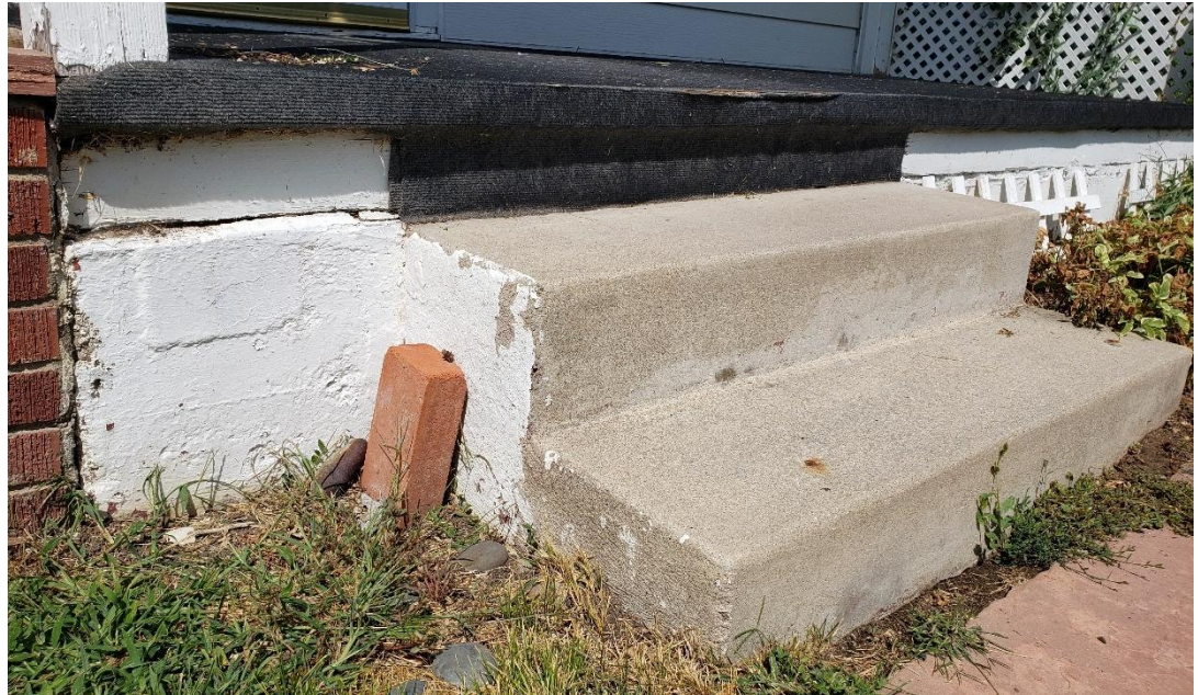
Concrete deck foundation, wood framing, and carpet over plywood with concrete steps.
