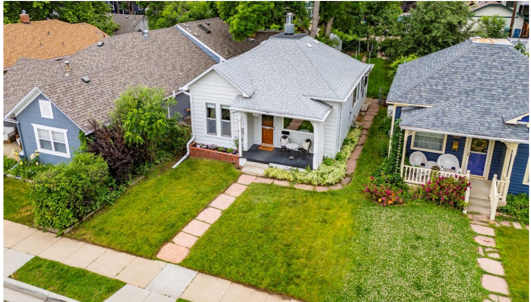
Looking west from above LaFarge Avenue.
