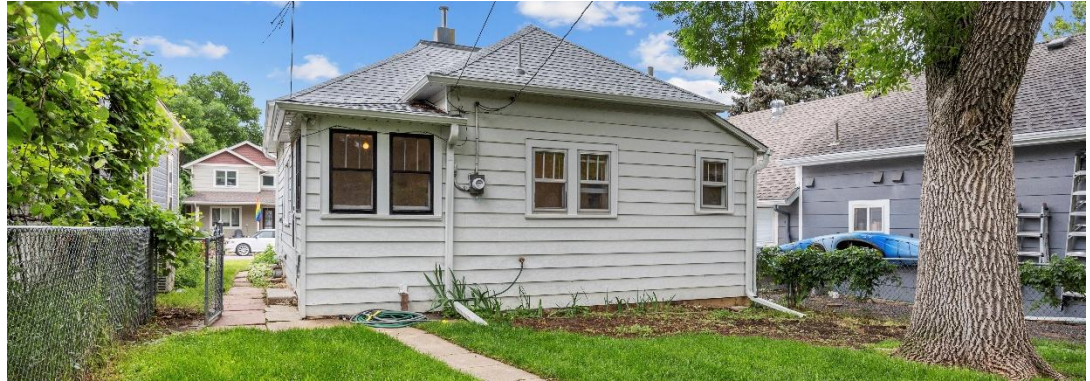
Grade is highest at the northwest corner of the house where finish materials are in contact with grade.
