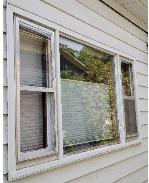
Replacement windows and aluminum storm windows.
