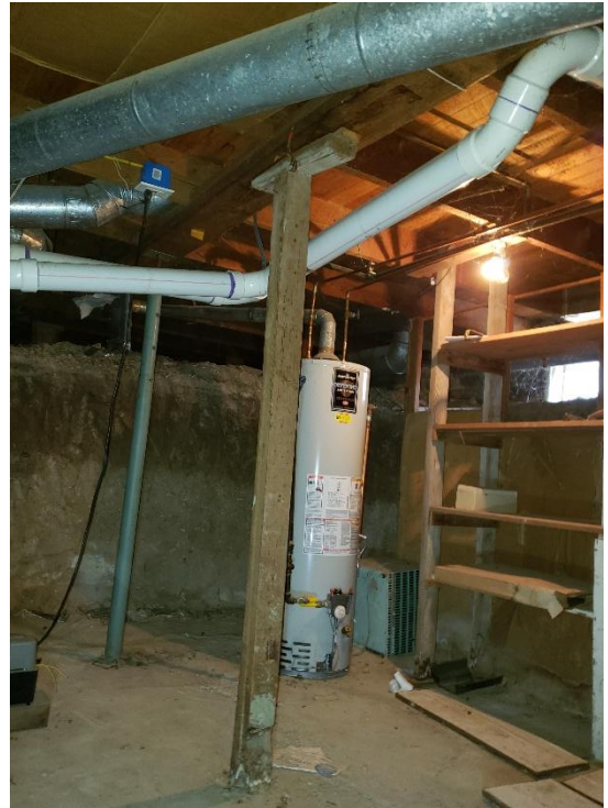
Wood and steel columns bear on the concrete slab floor.
