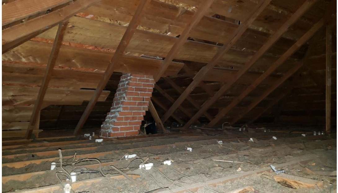
Remnants of a brick chimney above the kitchen seen in the attic.
