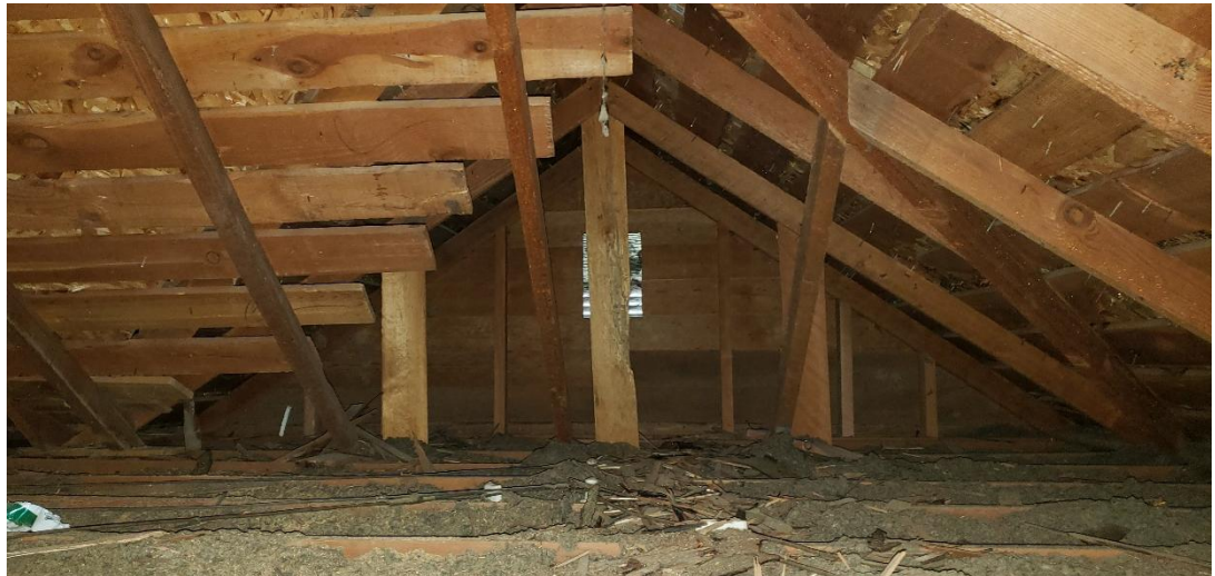
Gable end wall seen in the attic.
