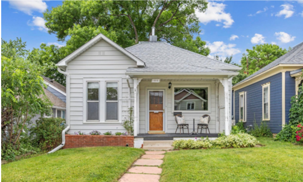
Street view of 1013 La Farge Avenue (July 2025, Courtesy of Ires ColoProperty)
