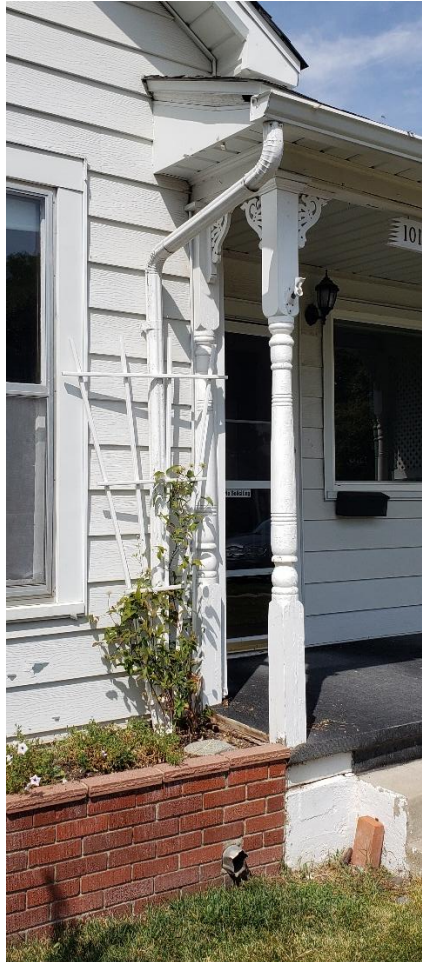
Round downspout buried in brick planter.
