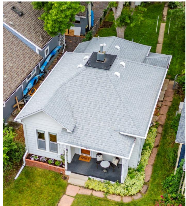
Asphalt roofing on the entire house with mushroom style vents.
