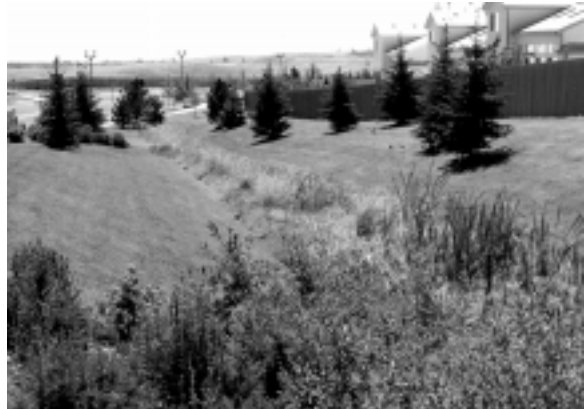
... USE GRASSY SWALES WHEN POSSIBLE AND DESIGN ALL ON-SITE DRAINAGE AND DETENTION FACILITIES WITH ATTRACTIVE, YEAR-ROUND SITE FEATURES AND AMENITIES.
