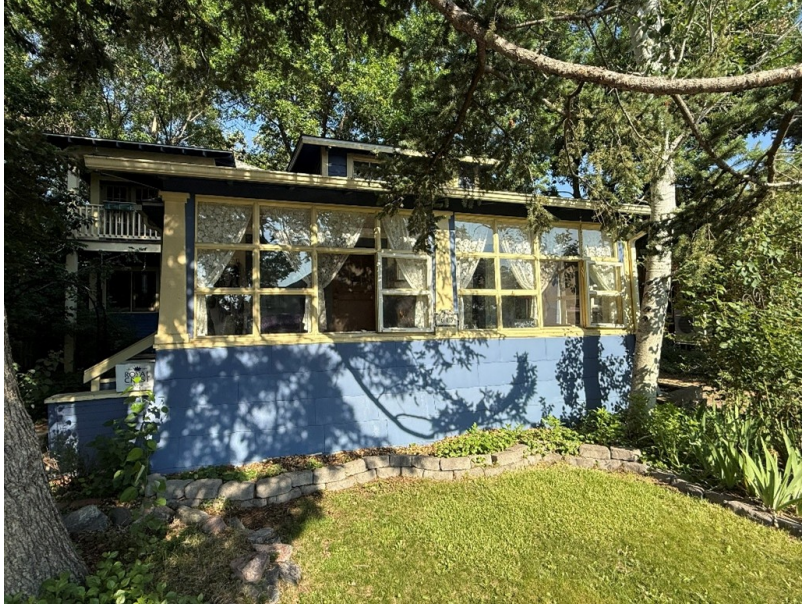
Photo 4 of Porch Windows, 2026
