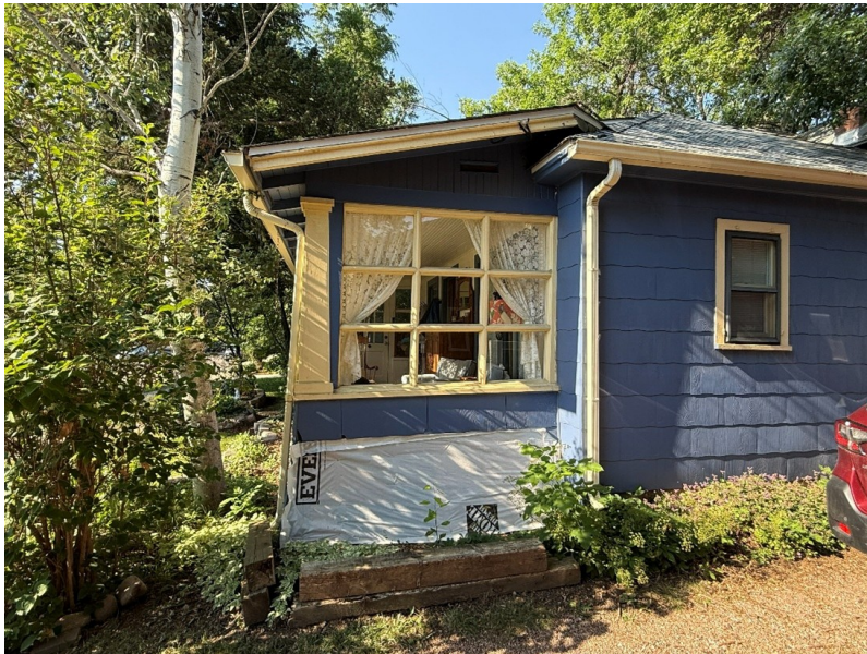
Photo 5 of Porch Windows, 2026
