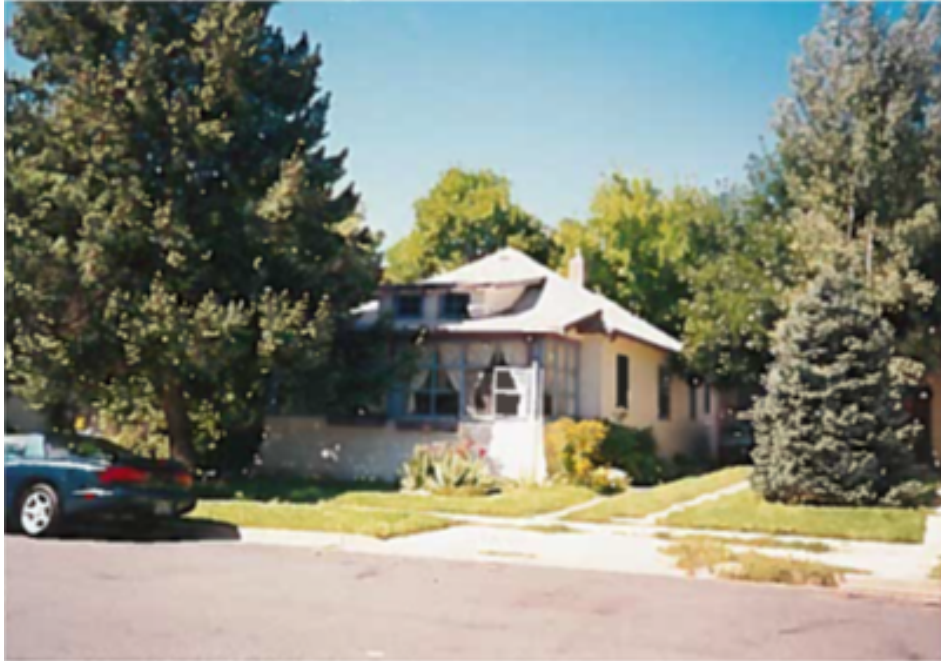
613 Grant – Prior to 1998 addition
