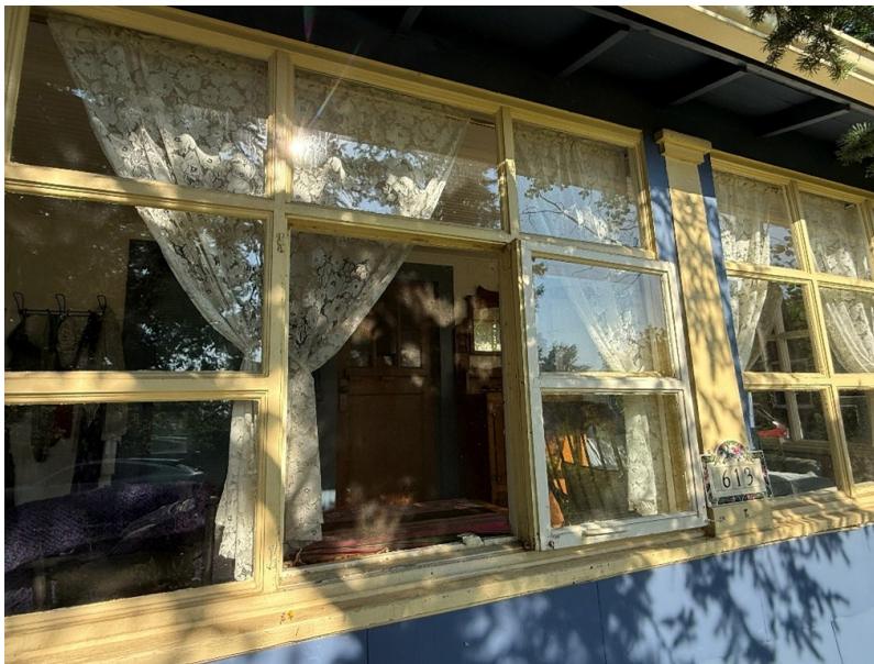
Photo 3 of Porch Windows, 2026
